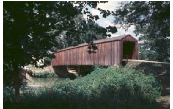
The covered bridge at Bollinger Mill State Historic Site in Bufordville.
