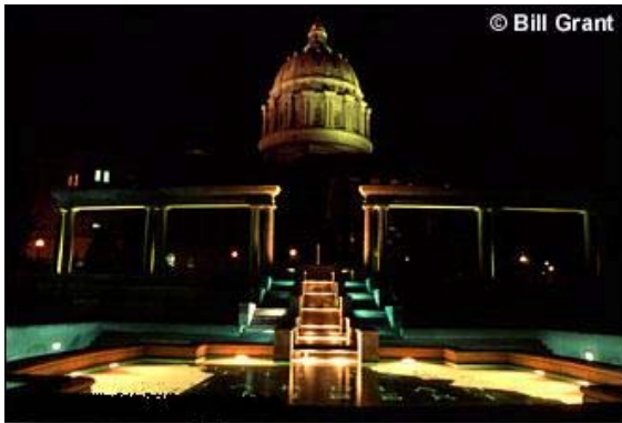
The All Missouri Veterans Memorial at the Missouri State Capitol features a limestone colonnade, terraced waterfall, reflecting pool, and eight black marble posts forming a path called the “Veterans Walk.”
