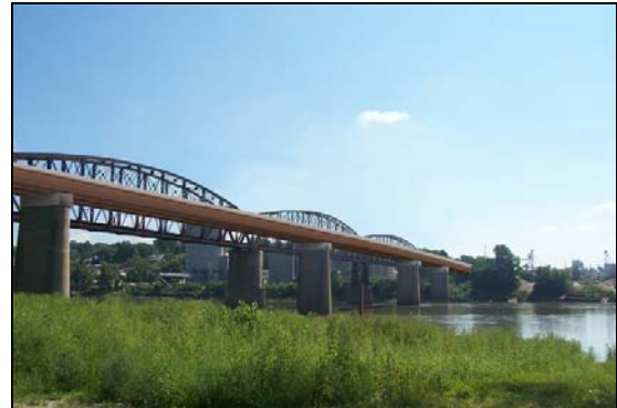
Glasgow Bridge – After Rehabilitation
