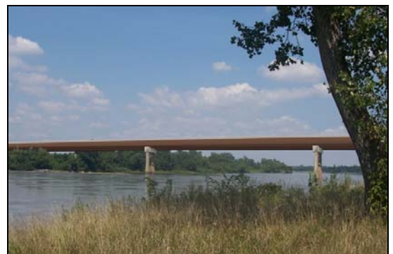
Miami Bridge – After Rehabilitation
