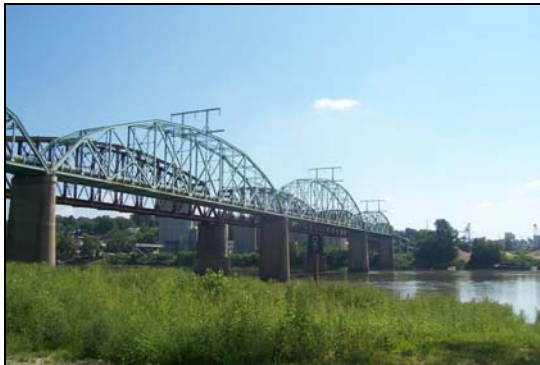
Glasgow Bridge – Current Condition
