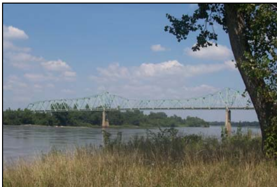
Miami Bridge – Current Condition
